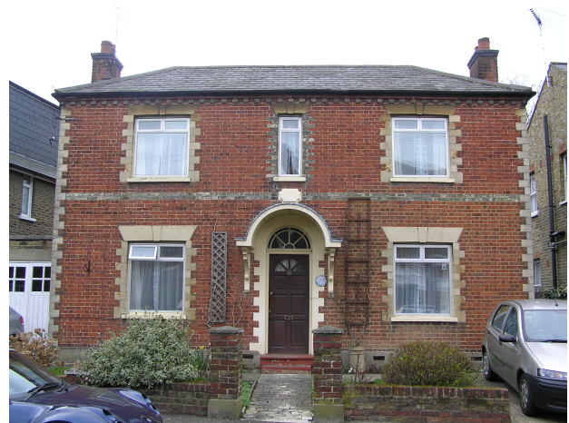
Picture 1.16 Victorian red stock brick and slate roofs
